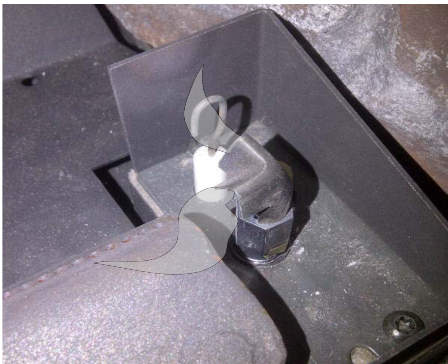
Figure 24. Correct Burner & Pilot Shield Placement (Q1LI Shown but similar to Q3LI)
